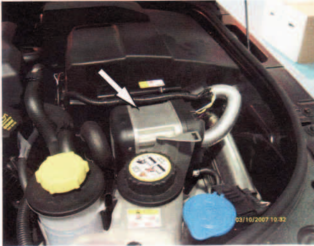
Photo 1 Showing top of Webasto (FFBH) directly in front of the battery cover
