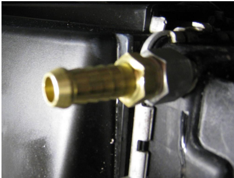
10. Fitting screwed in place with thread sealant
